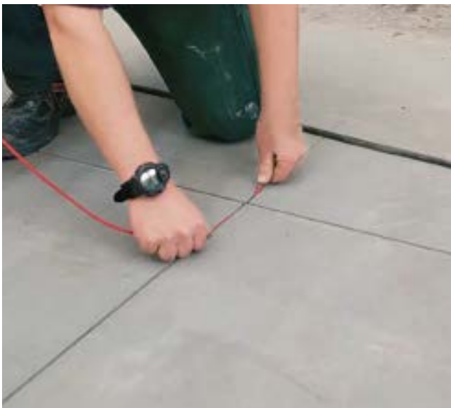
Fig. 13 Inserting the cable.
